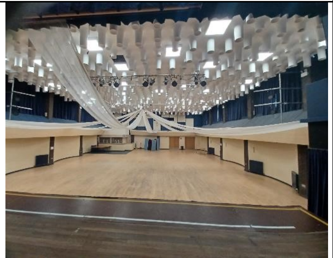
Theatre fixed ceiling – pre removal
