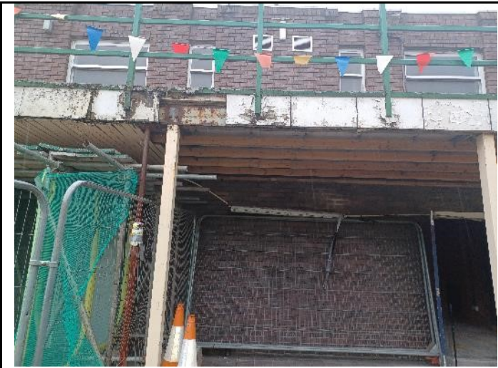
External canopy, corrosion of steel beam and support propping
