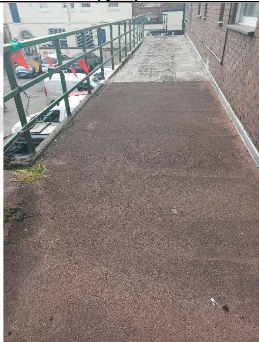
External (part) view of external covered walkway canopy asphalt/felt roof
