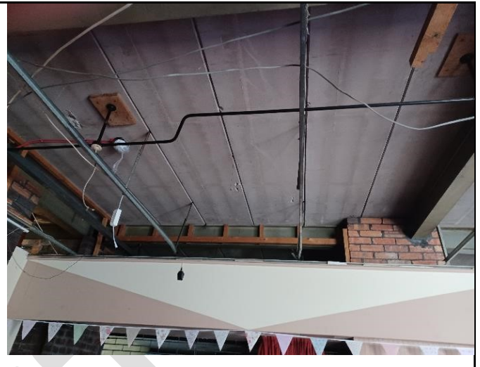
Social Area ceiling removed and fixing/ghosting to planks
