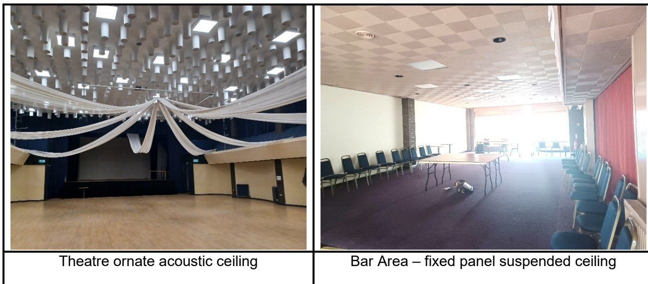
Figure 11 - Civic Centre - fixed/concealed ceiling example. Source Author
