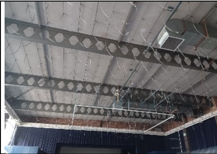
Theatre - Post ceiling removal – showing castellated beams and fixings to planks.
