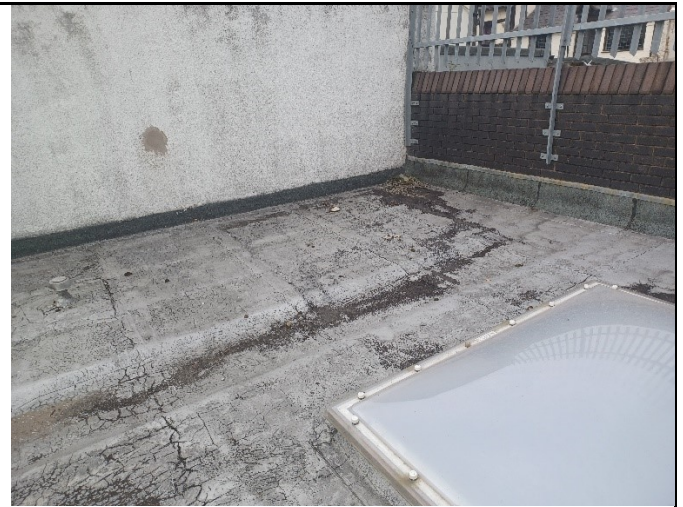
Library rear Asphalt flat roof
