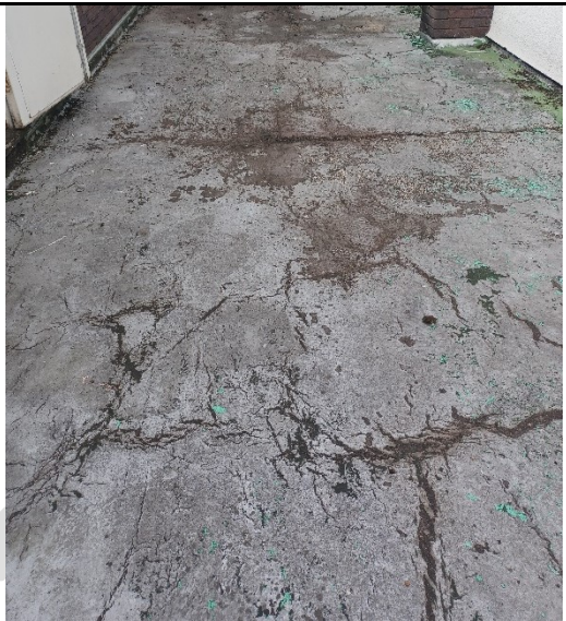
External view of internal covered walkway canopy asphalt roof
