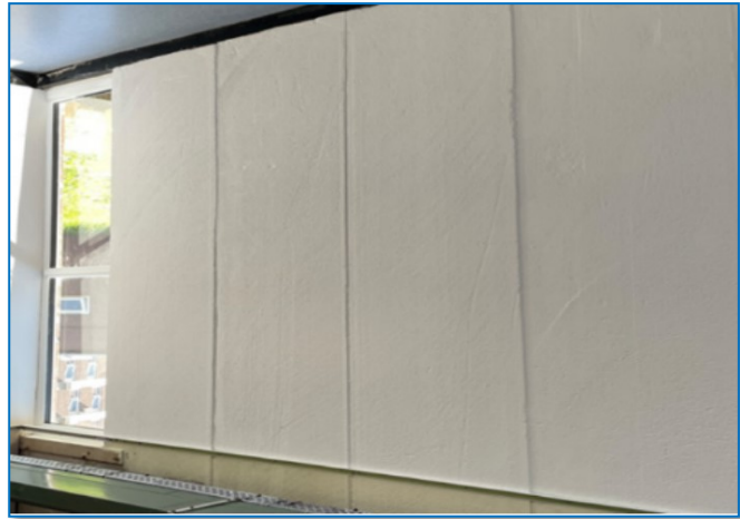
Figure 28 - RAAC Wall Construction. Source DfE (2023)
