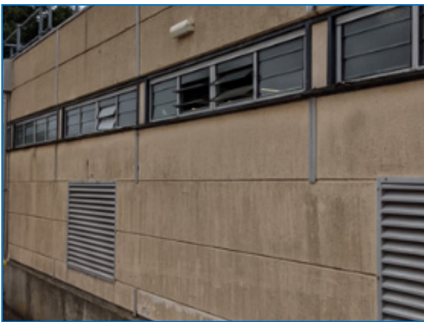
Figure 28 - RAAC Wall Construction. Source DfE (2023)
