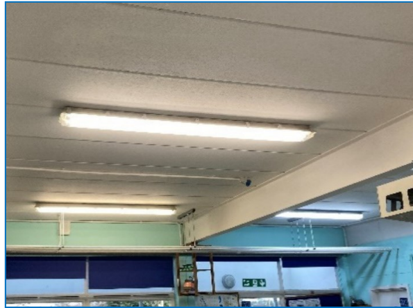
Figure 27 - RAAC roof/Floor. Source DfE (2023)
