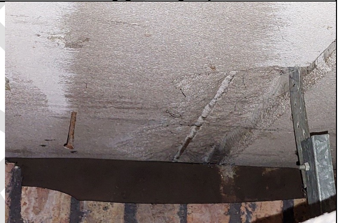
Social Area ceiling removed and fixing/ghosting to planks
