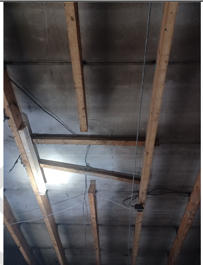
Timber beams to underside of RAAC planks
